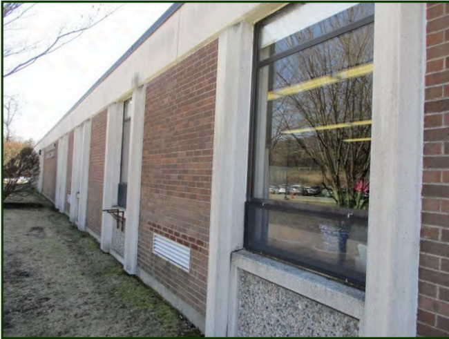
Original Window Full View
